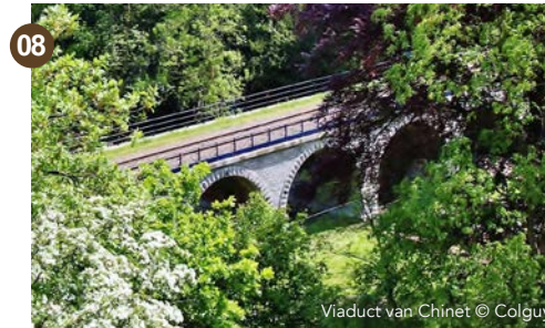
Viaduct van Chinet © Colguy
