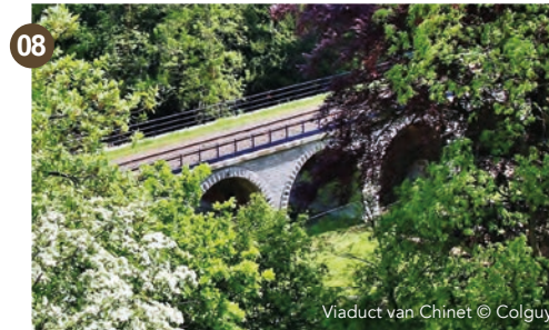
Viaduct van Chinet © Colguy
